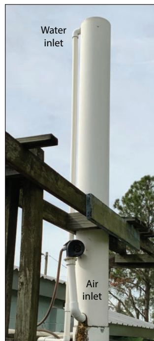
Figure 3. A degassing unit on a Florida ornamental fish farm. The pipe on the left brings water to the top of the unit, and the air pump at the bottom supplies air into the unit. Water drops down the unit as air is pumped upward, creating a countercurrent exchange and drawing unwanted dissolved gases from the water.
