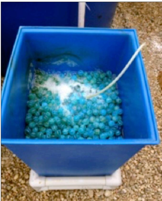
**Figure 9.** Biofilter tank.
