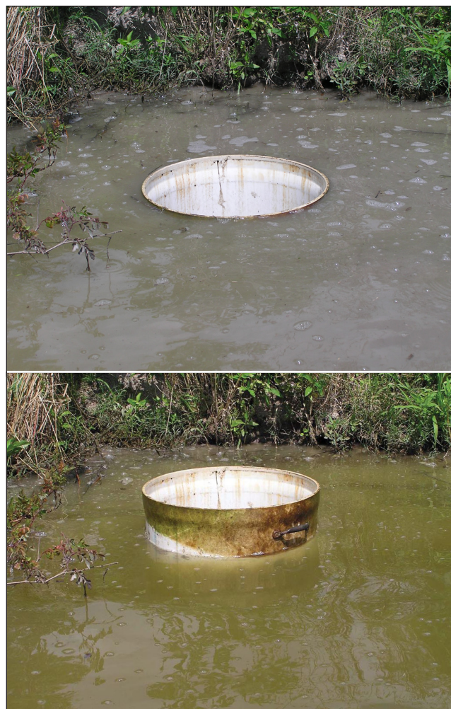
Unintentional effluent releases from warmwater aquaculture ponds can be reduced by increasing pond storage capacity 4 to 8 inches to capture excess precipitation.
