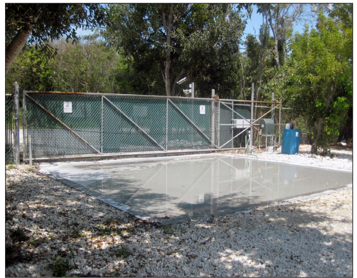
Figure 6. A drive-through disinfection area, consisting of a shallow area filled with disinfectant, to disinfect vehicle wheels.
