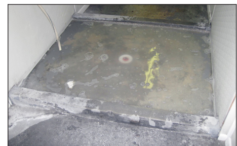
Figure 3. Concrete footbath built into the floor of the hallway.
