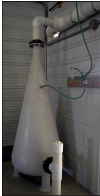
Figure 4: An oxygenation cone commonly used in pure oxygen systems.
