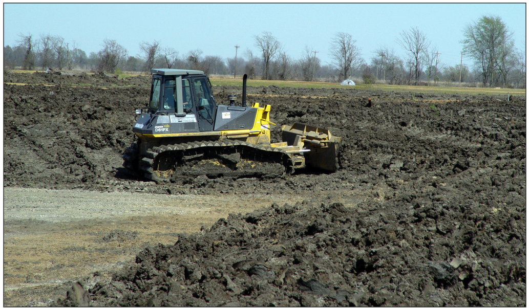
Figure 3. Bulldozer constructing levees.
